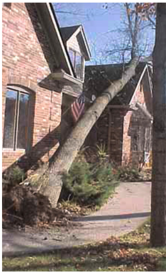
This tree looked healthy to the untrained eye; however it had a cavity in the trunk and was toppled in a wind storm.
